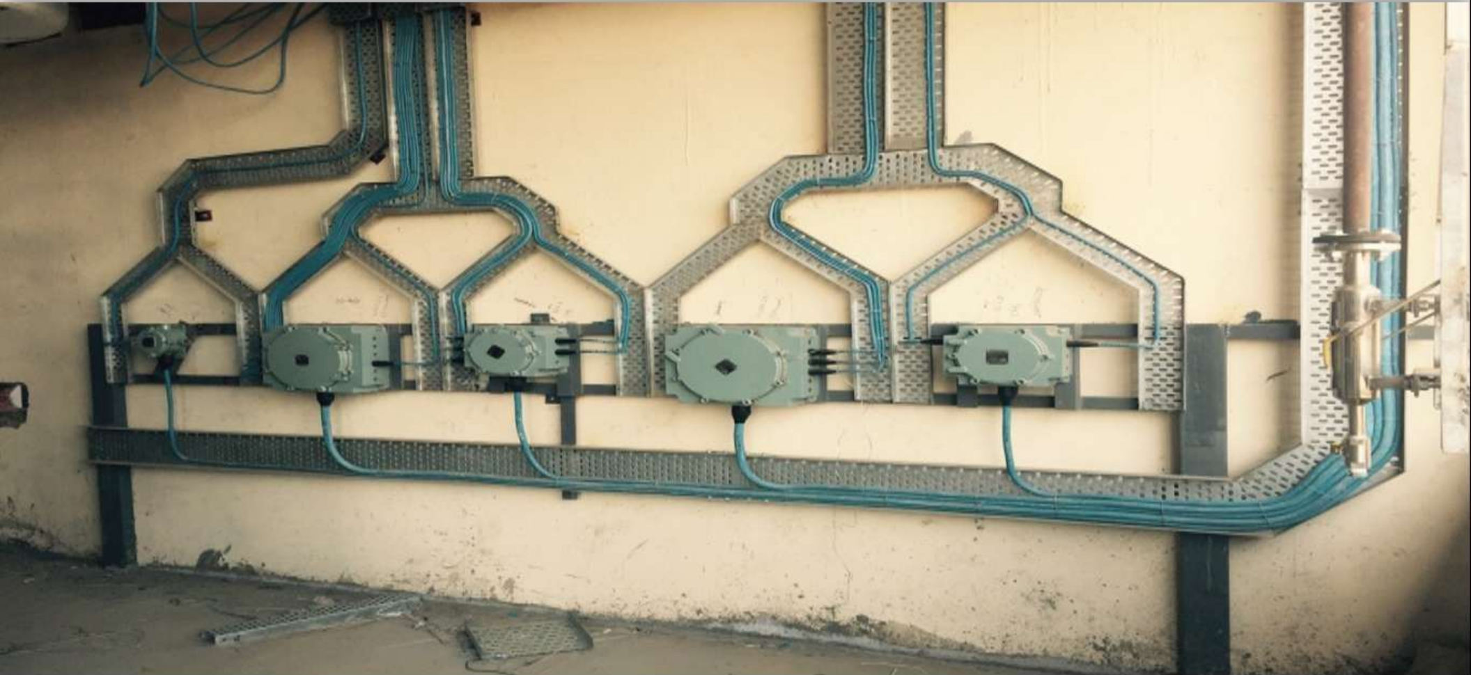
Perforated Type Cable Tray for Instrumentation
