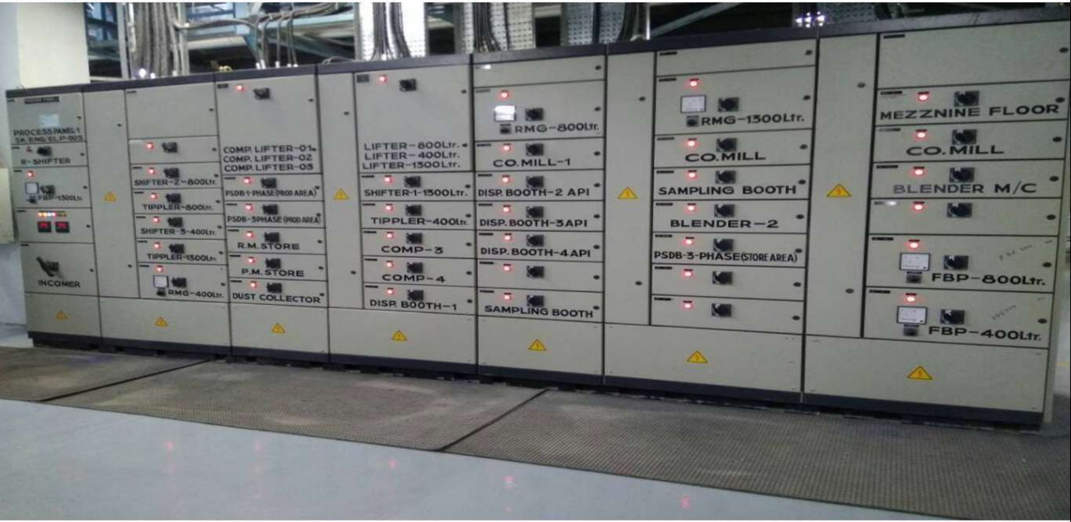
Nomenclature to Each Feeder on LT Panel
